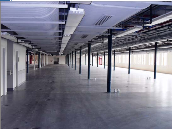
Building 16—1st Floor
